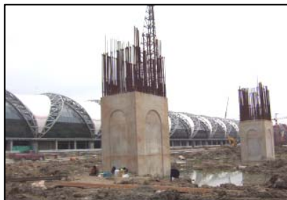
Couplers of elevated frontage road
