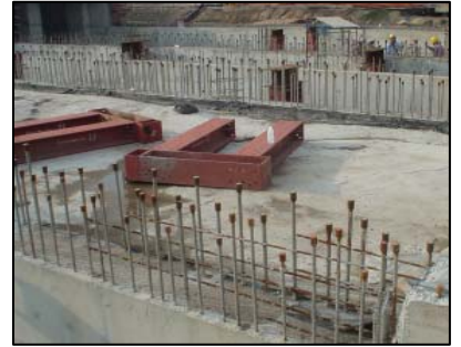
Couplers in beams
