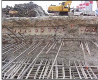
Couplers in diaphragm walls
