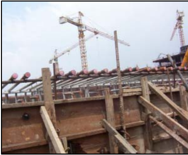
Couplers in construction joints
