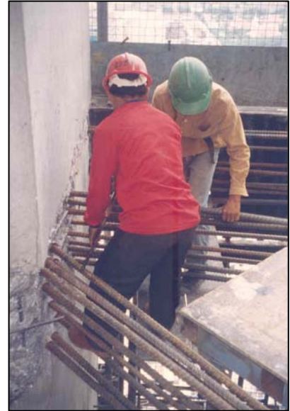
Beam to column connection
