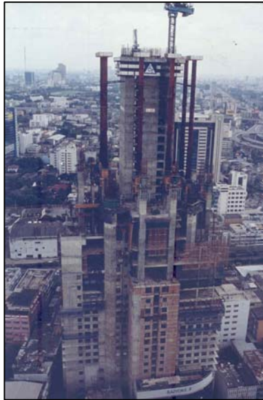
Construction of upper core wall and lower floors
