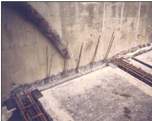
Starter bars after removal of the box
