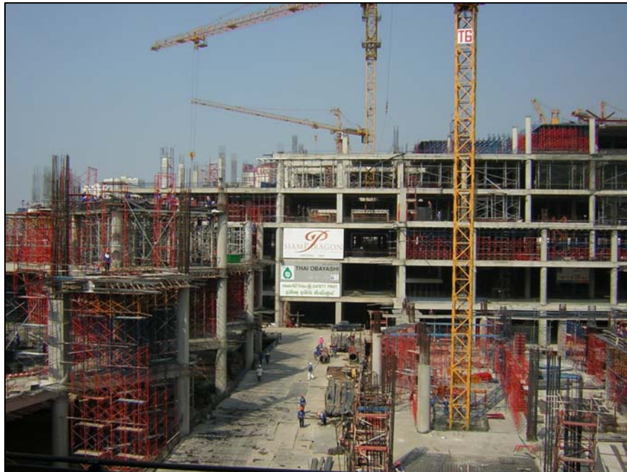
Overall site view
