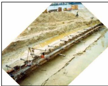
Retaining wall completed
