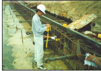
Preparative of retaining wall
