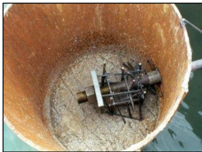
Preparation of anchoring pile
