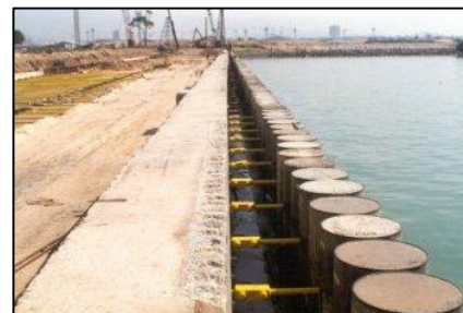
Load full completed
