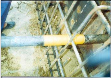
Preparation of connection to mainland
