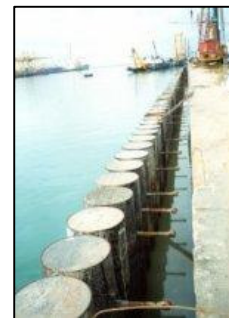
Anchoring piles connected
